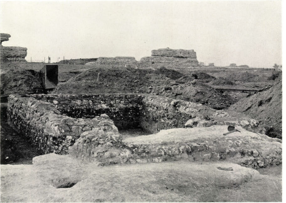
FIG. 2. The building on site IV, looking west, p. 32
