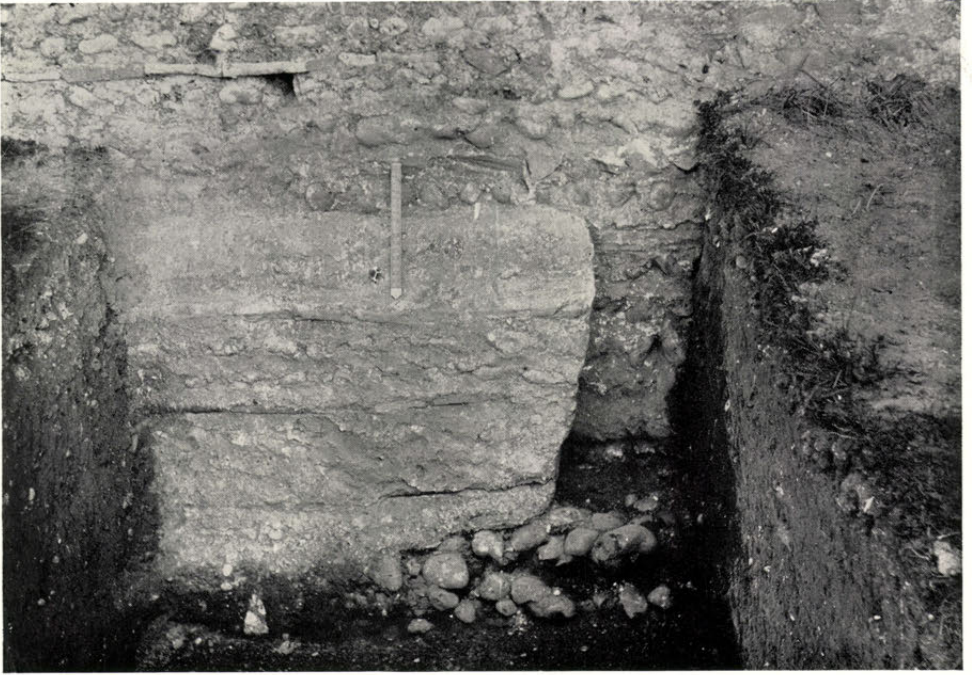
FIG. 1. End of the moulded plinth on the inner face of the north wall of the Saxon Shore fort. Section 37, p. 53
